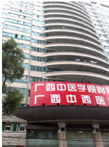
Image: Ruikang Hospital #2, Nanning, China.
